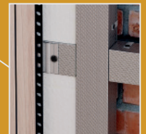
mounting clip is installed into a slot for tongue at \leq 600 mm pitch, and latched to the guide via a tapping screw
